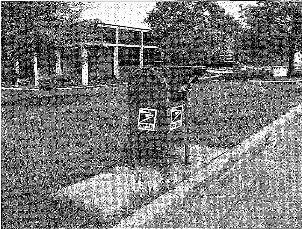
8800 NW 112 th Street – looking northwest – deterioration of street furniture (mailbox) and concrete pad
