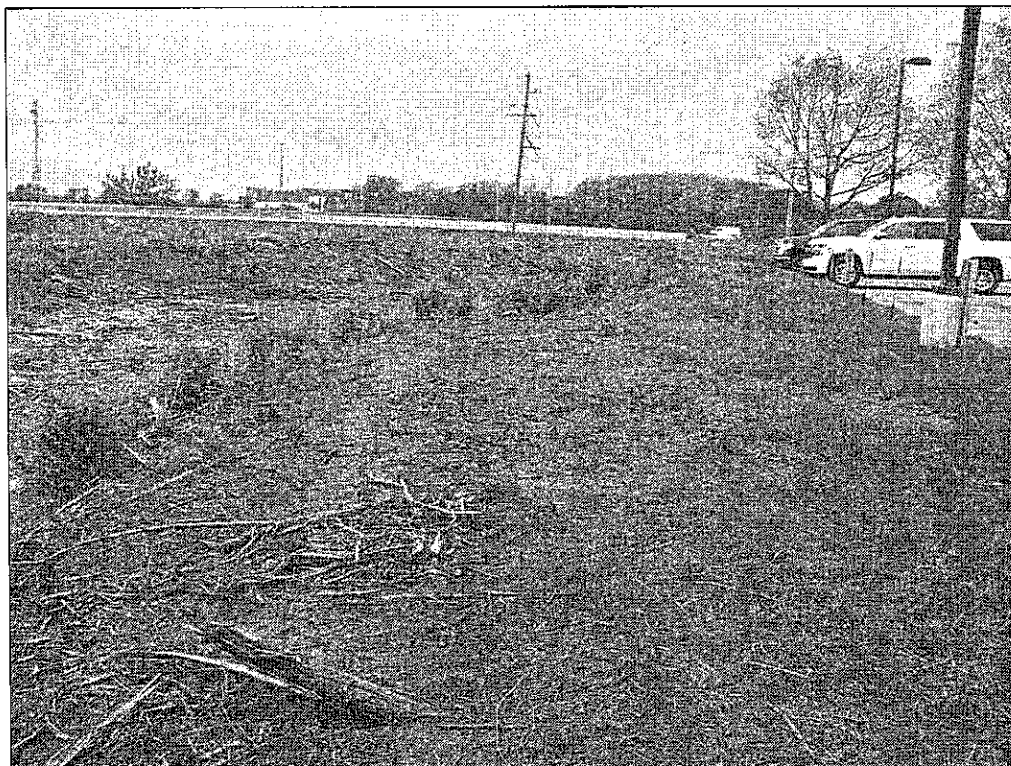
Parcel APN 17-6.0-23-000-000-036.000 – looking southwest – lack of landscaping; debris
