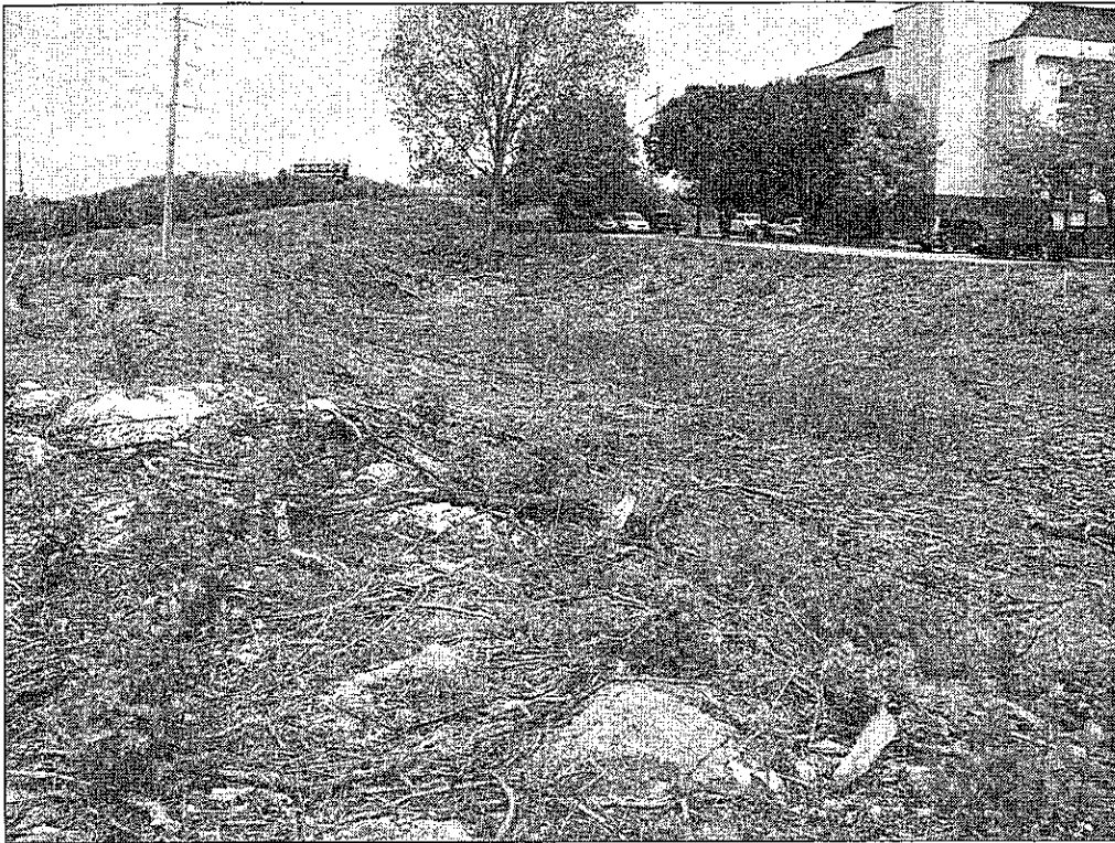
Parcel APN 17-6.0-23-000-000-036.000 – looking northwest – deterioration of drainage improvements
