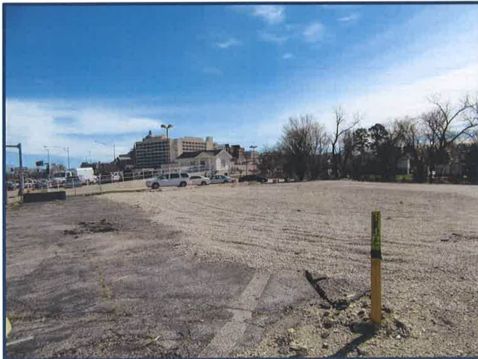
Deteriorated asphalt on the Southeast Tract
