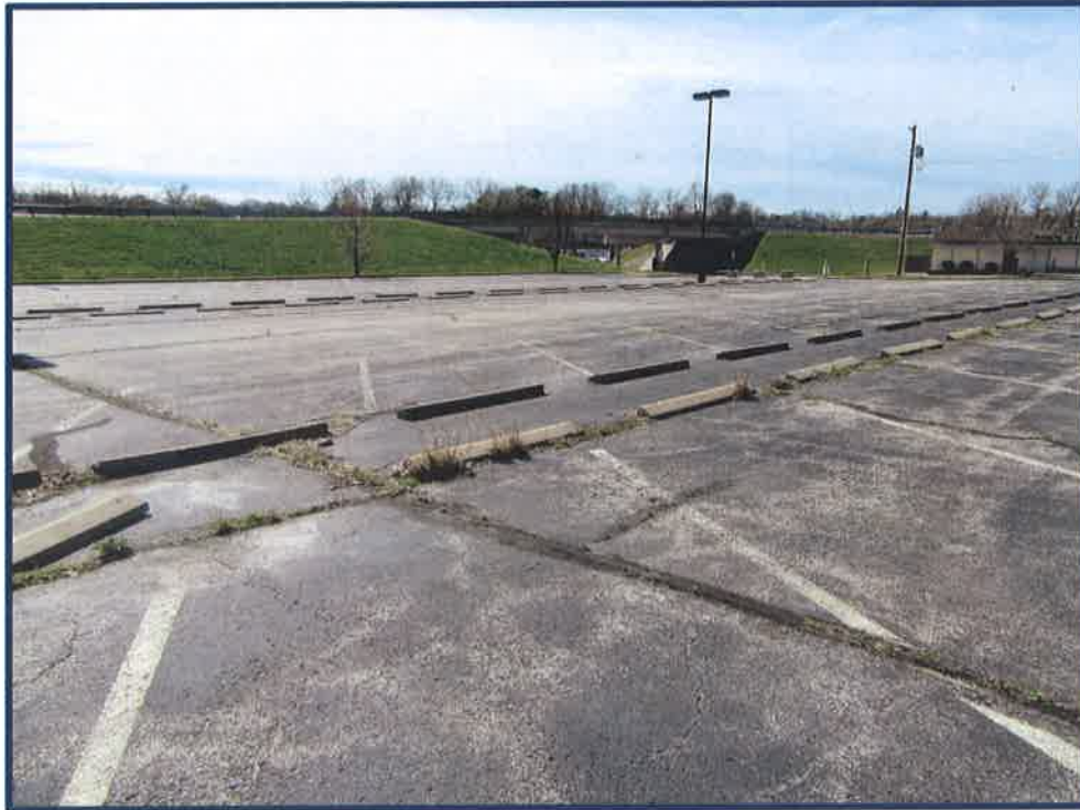
Deteriorated asphalt, weeds growing in parking area on the Southwest Tract
