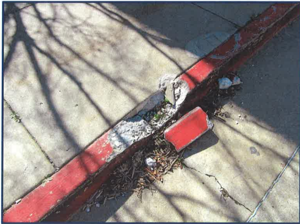
Crumbling curb near the entrance area
