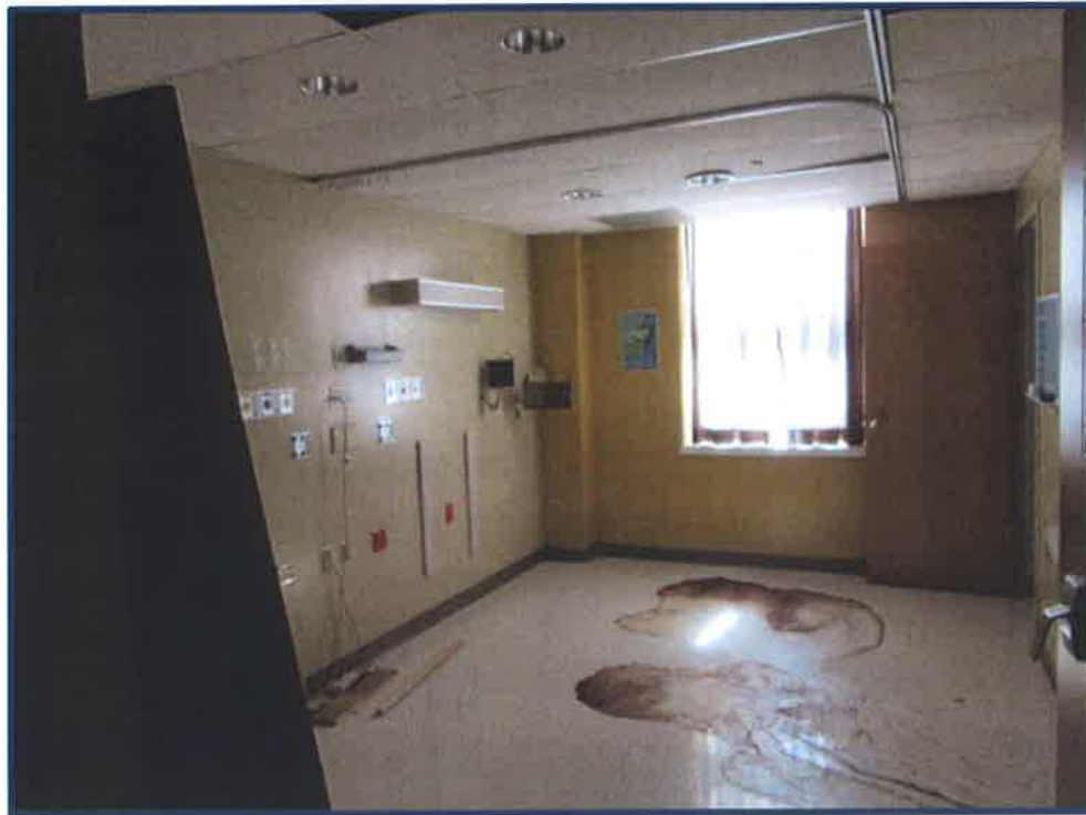
Floor stain due to leaking roof is considered to be unsanitary.
